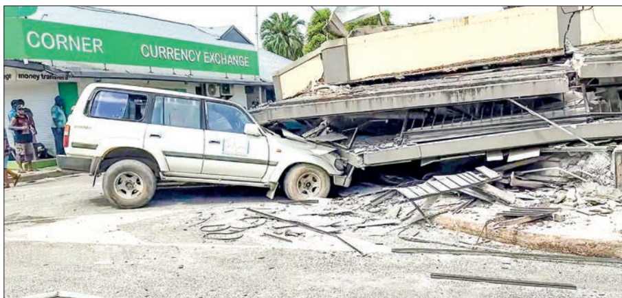
This screengrab taken from handout video footage posted on the Facebook account of Michael Thompson on 17 December 2024 shows people inspecting a damaged car trapped underneath a collapsed building in Vanuatu's capital Port Vila after a powerful earthquake hit the Pacific island. PHOTO: MICHAEL THOMPSON / FACEBOOK ACCOUNT OF MICHAEL THOMPSON / AFP
